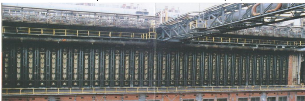
Full View of Coke Oven
